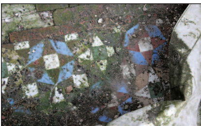
▲ Fig. 10 The tile floor in the Glenlair House foyer.
